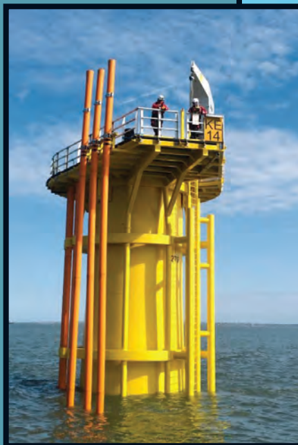
Seaproof's J-tube interface.
